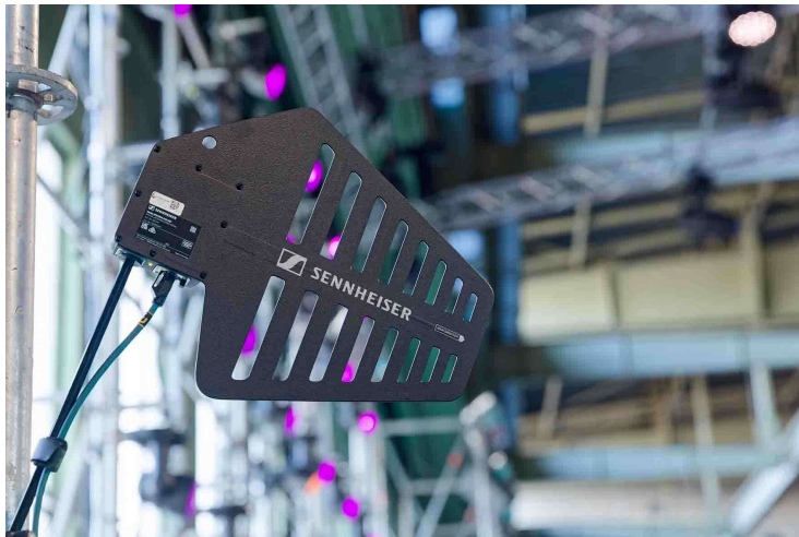
Eight Spectera DAD antennas were installed in Hangar 4
