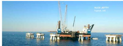
The overall fleet is now composed of two 1,100-ton capacity self-elevating platforms fitted with 250-ton cranes, two backhoe transport barges.
