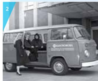
1 The T2 Elektro Transporter had to be connected to a charging unit for several hours to charge the batteries. Alternatively, the entire set of batteries could be changed.
