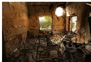
System identifier: MSF154407 Title: Kunduz Hospital, Afghanistan, October 2015 Photographer / cameraman: Victor J. Blue Countries: Afghanistan Description: An interior view of the MSF Trauma Centre, 14 October 2015, shows a missile hole in the wall and the burnt-out remains of the building after a sustained attack on the facility in Kunduz, northern Afghanistan..
