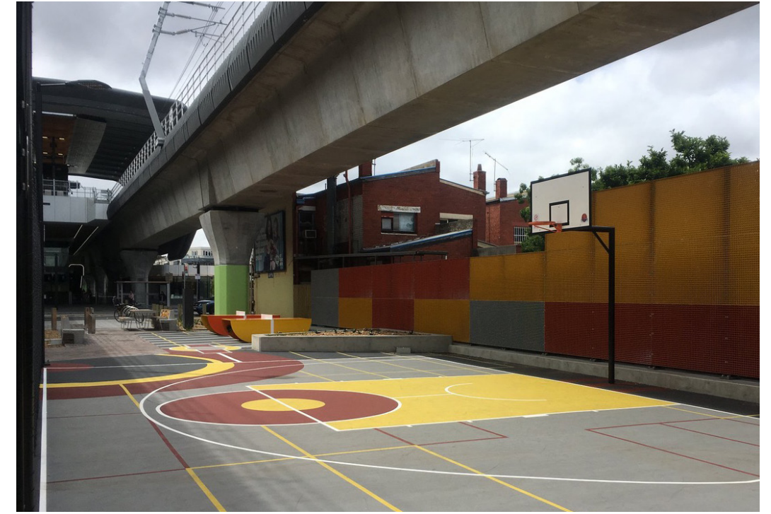
The Clayton Road Community Space, Clayton
