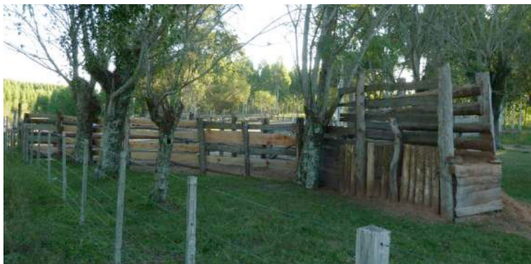
Loading ramp at collecting station of Bardanca.
