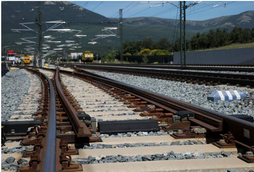
High speed track in Spain ©Thales
