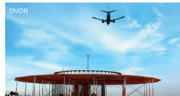
Until now, 9 wind turbines per 60° sector could be installed in a radius of seven kilometres around a DVOR. **Now, thanks to the new dynamic calculation mechanism, there is room for up to 18 wind turbines per sector of 60°.** This enables skeyes to contribute to a sustainable future.
