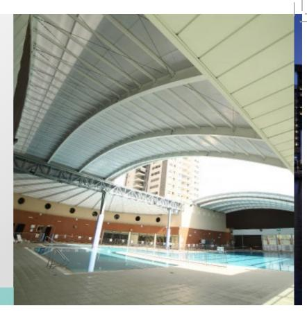
The roof of the Swimming Pool in Ramle is made out of an integrated system of fixed and moving multiwall polycarbonate sections.
