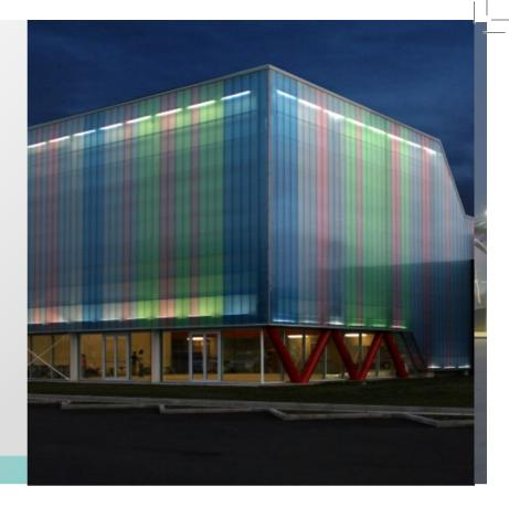
The building was constructed by using two materials: black steel panels as well as **coloured and translucent polycarbonate**. It serves as a multipurpose center for sport.
